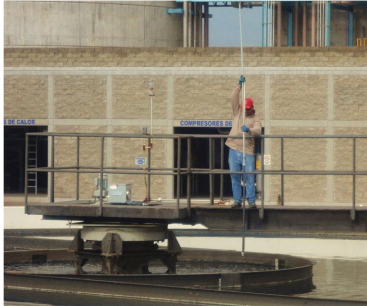
Figure 2.9 An operator at a WWTP in Mexico uses a “sludge judge” to measure the clarifier’s blanket depth.
